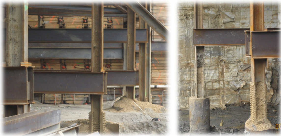
Figure 2 & 3: Bracing at the M Street Ramp
